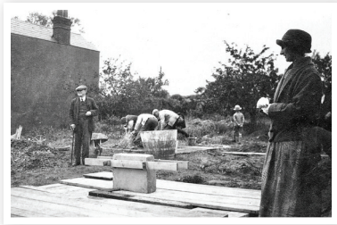
May 1924 – The Cornerstone (foreground) ready to be laid
